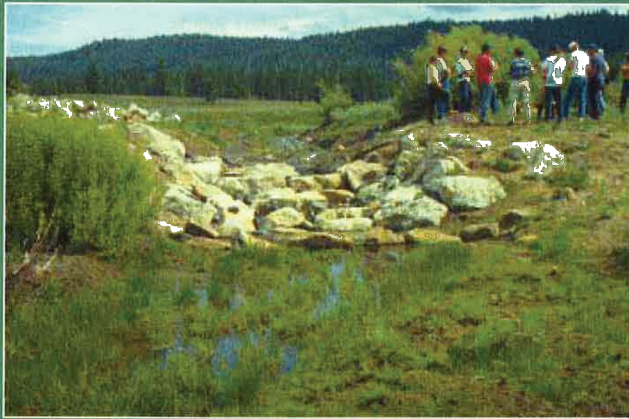
Depicted above is a loose rock gully control structure being used to stop headcutting up into the meadow. Note that the rock structure is well keyed into the banks and channel bottom.
