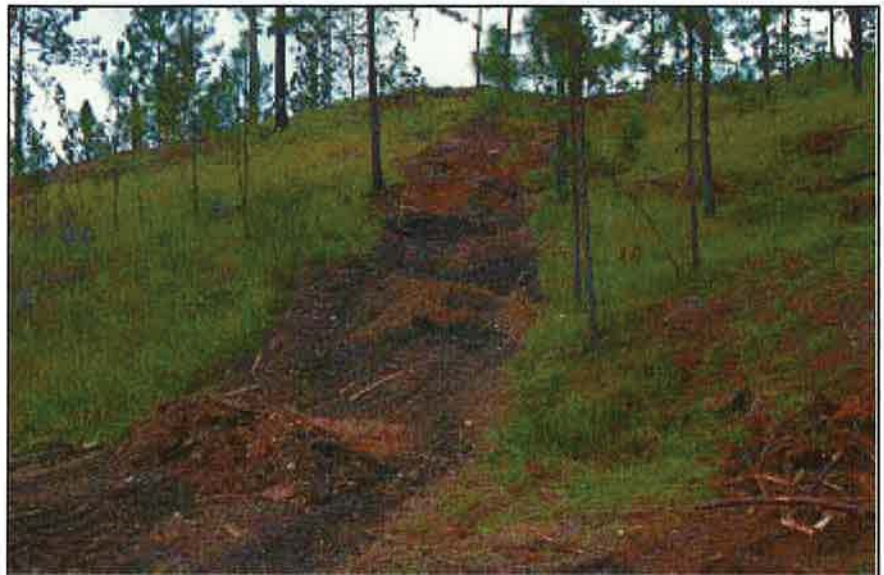
Photo 3.8 Stabilize skid roads and trails after use with water bars and apply a ground cover or other erosion control measures.
