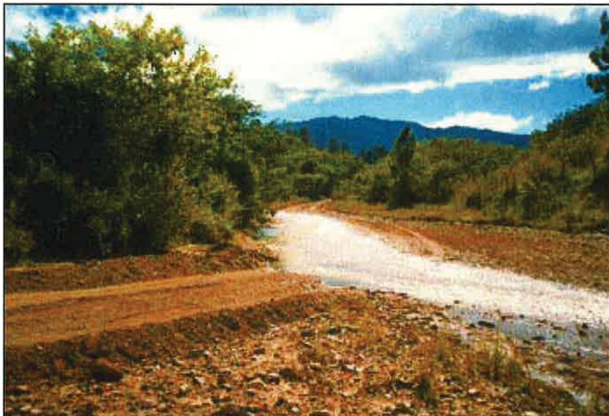
Photo 7.8 Avoid natural drainage crossings that are broad and that are not perpendicular to the drainage. Stay out of the stream! This broad channel is a good site for a vented ford.
