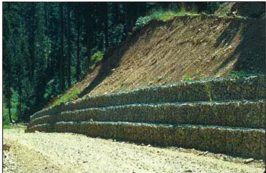
Photo 11.9 Gabions are a commonly used type of low gravity retaining structure because they use locally available rock and are relatively inexpensive.
