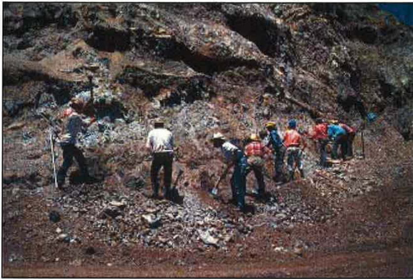
Photo 12.9 Develop quarries and borrow sites (materials sources) close to the project area whenever possible. Either hand labor or equipment may be appropriate, depending on the site conditions and production rates.
