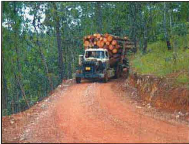
Photo 4.5 A stable logging road with aggregate surfacing. Use road surfacing materials as frequently as possible to reduce erosion and improve the roadbed structural support and rider comfort.
