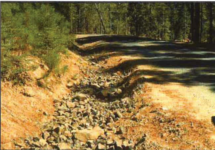
Photo 13.5 A roadside ditch armored with graded rock (riprap) for erosion control.
