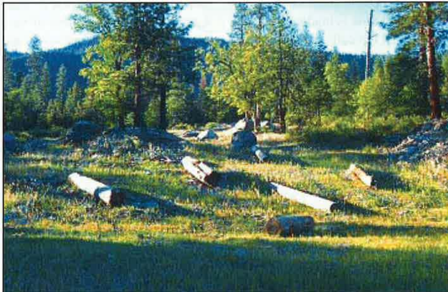
Photo 12.12 A reclaimed and revegetated borrow site. Reshape, drain, plant vegetation, and rehabilitate borrow pits and quarries once the usable materials are removed and use of the area is completed.
