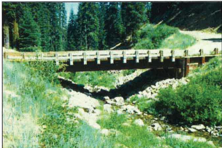
Photo 10.6 Here is a well built treated timber bridge with good streambank protection and adequate span to minimize stream channel impacts. The freeboard is marginally adequate.
