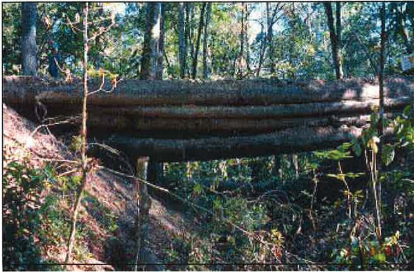
Photo 10.2 A bridge structure typically offers the best channel protection by staying out of the creek. Use local material for bridges as available, considering design life, cost, and maintenance. Inspect bridges regularly, and replace them when they are no longer structurally adequate.
