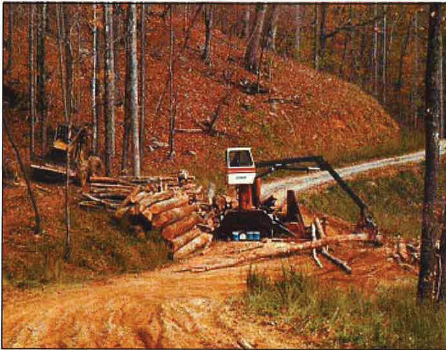
Photo 3.7 Locate logging roads and landings away from SMZ's and water courses. Keep the roads and landing areas small and efficient.
