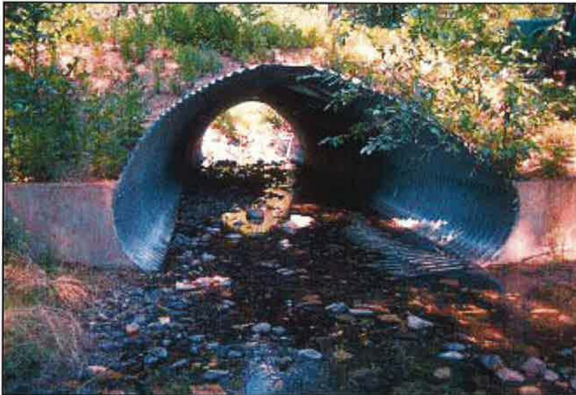
Photo 8.7 Use structures with natural stream bottoms, such as arch pipes, bottomless arches, or concrete box culverts, to promote fish passage and minimize impacts to the stream.
