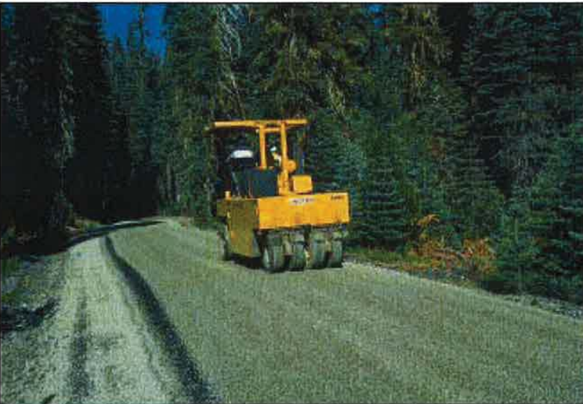
Photo 12.8 A chip seal road surface being compacted. A variety of surfacing materials can be used, depending on availability, cost, and performance.
