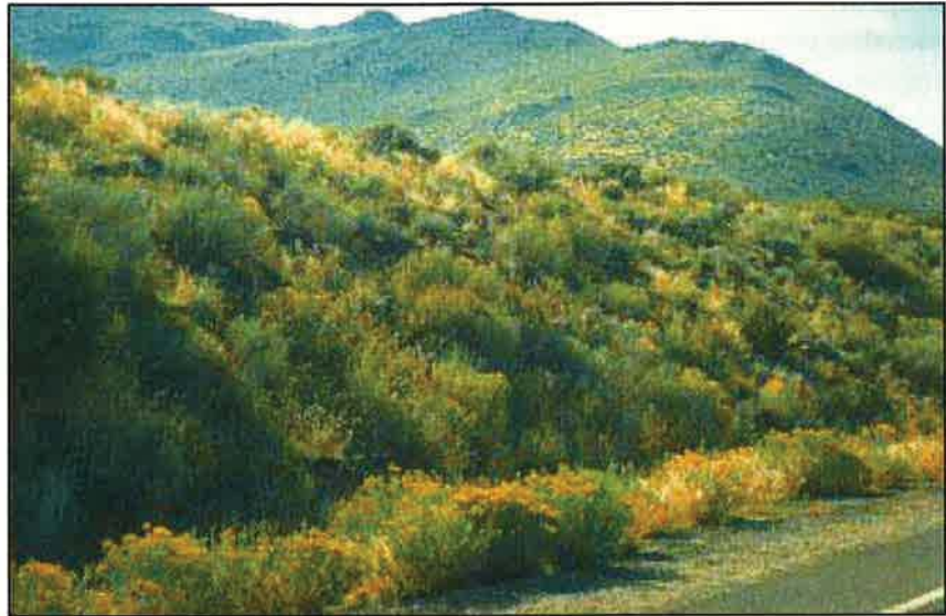
Photo 11.3 A well-stabilized cut slope, with about a 1:1 slope, that is well covered with vegetation.
