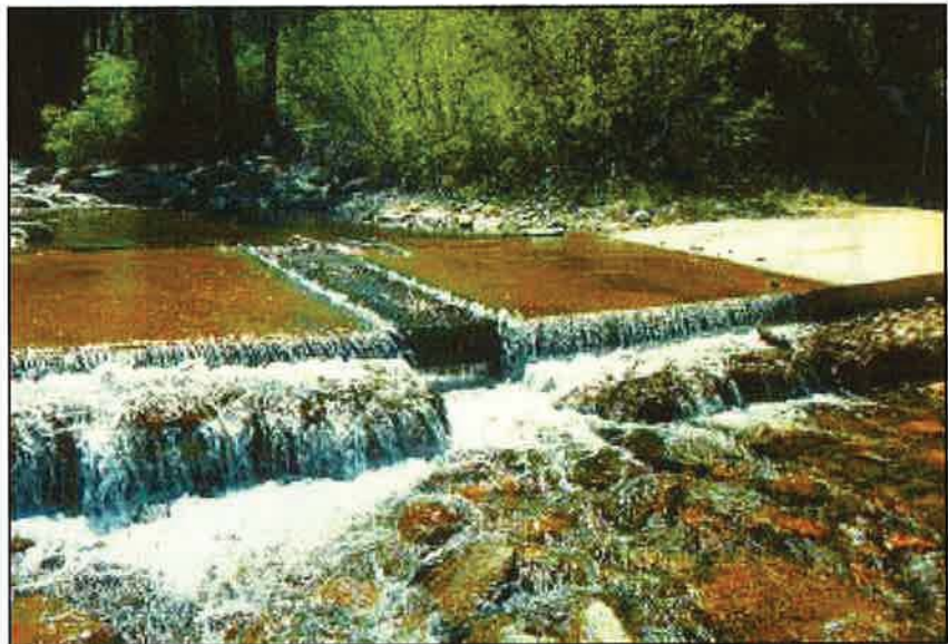
Photo 9.4 Use vented fords with pipes or openings to keep traffic out of the water most of the time, minimize traffic delays, and allow for fish passage. Note the downstream scour protection with gabions and rock.
