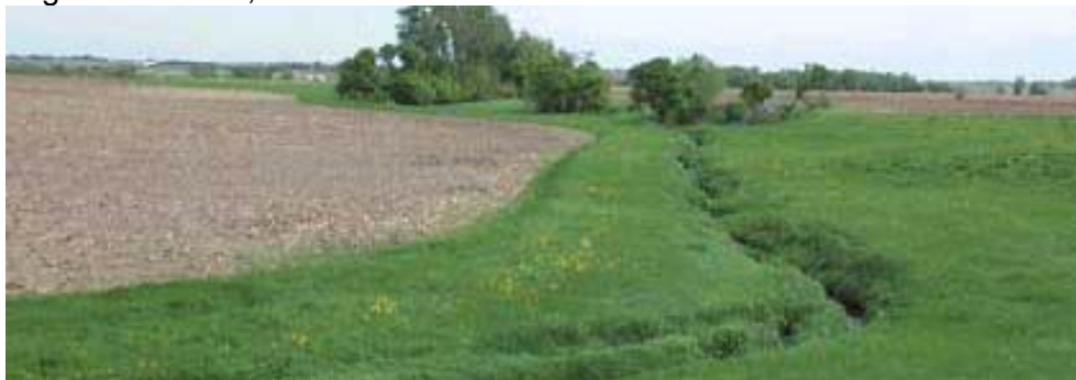
A 20-foot wide vegetated buffer strip between a creek and disturbed bare land. Source: Carleton College Seven-Mile Creek Watershed Project
