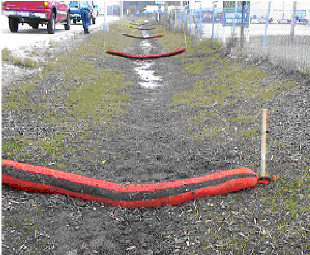
Compost Socks staked in place along a storm water swale. Source: Ohio Department of Transportation, 2008
