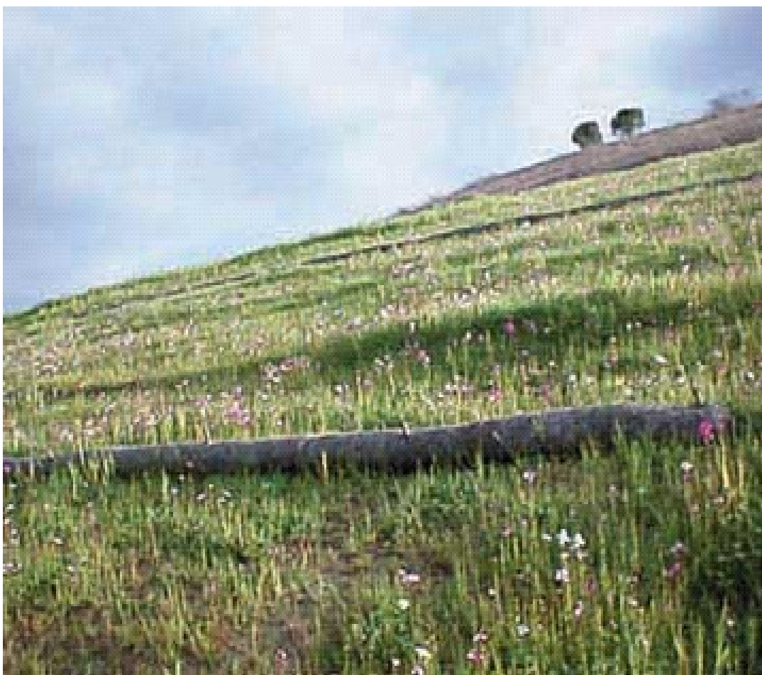
Fiber rolls along a newly-vegetated hillside. Note the disturbed slope at the top of the hill Source: EPA Storm Water Menu of BMPs, 2004
