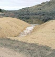
Following construction, the use of an erosion control mat, improves reclamation success.
