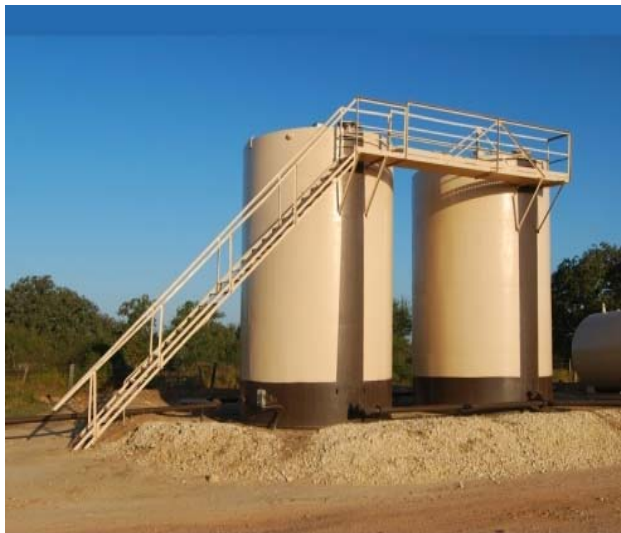
Twin 210 barrel oil tanks inside containment dike
