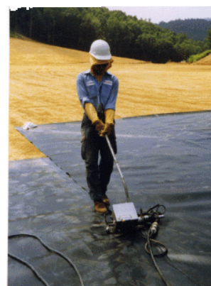
Joining the seam of a synthetic liner
