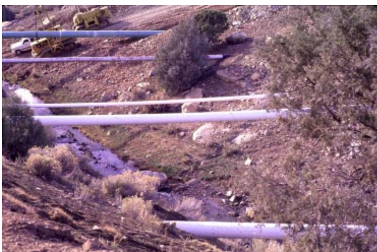
Aboveground pipelines, exposed and crossing a creek in Colorado. Note the size of the pipelines in comparison to the equipment in the background.
