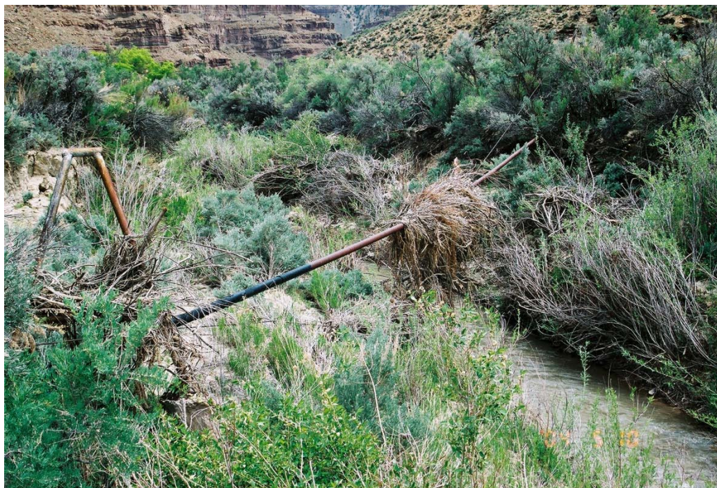
Figure 3. Although this pipeline crossed above the bankfull channel indicators, it was not high enough to escape more extreme floods.
