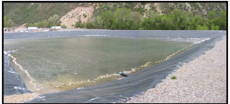
Encana’s “Middle Fork Water Storage Pond”: SUP for Storage, Processing & Material Handling of Natural Resources (for storage of produced water where adjacent tanks were used to separate hydrocarbons from water)
