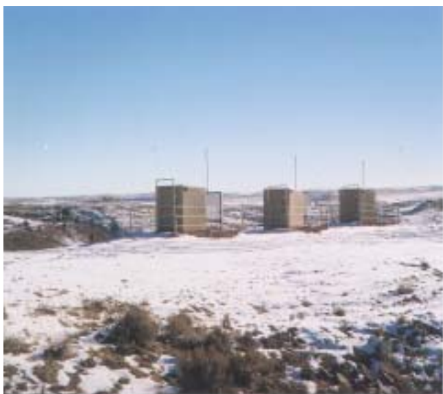
Three CBM wells finished with surface enclosures in the Powder River Basin
