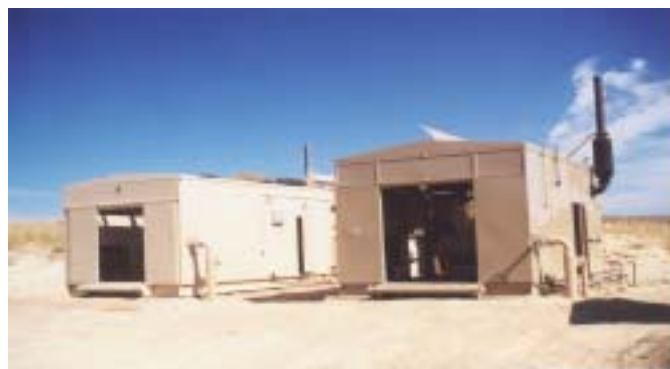
Photograph of typical CBM field compressor station
