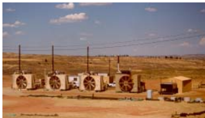
Typical sales compressor facility in the Powder River Basin, Wyoming
