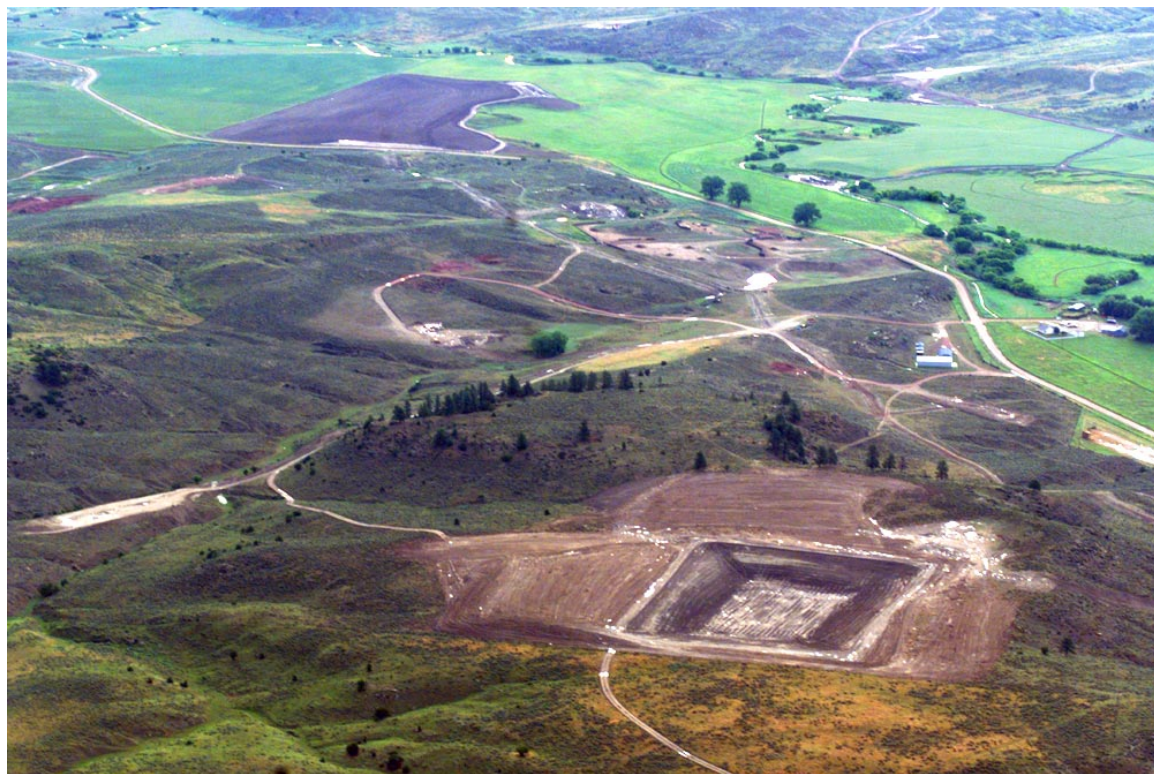
The construction of one reservoir in Wyoming's Powder River Basin for CBM-produced water containment. Wyoming already has over 1,000 reservoirs in place or permitted, and can expect thousands more over the life of the CBM play with at least 50,000 wells predicted by 2010 for the basin.
