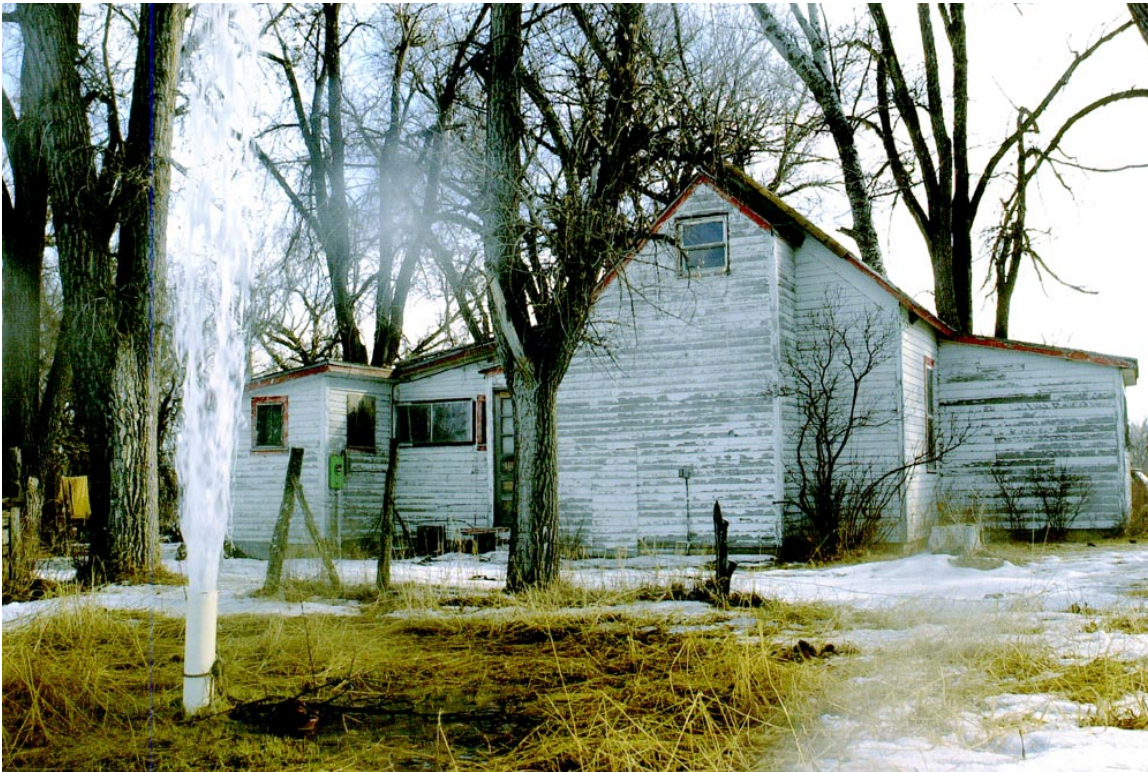
Methane from CBM wells can migrate through underground faults following the path of least resistance. Migrating CBM causes this previously capped water well to explode just feet from a Wyoming residence.
