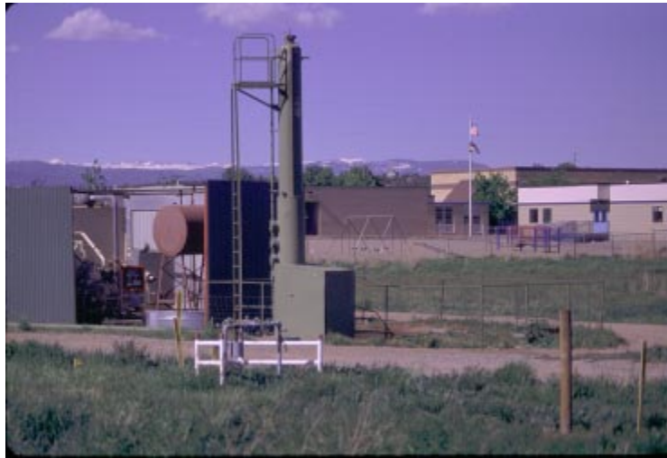
Wellhead compressor near an elementary school in Colorado.
