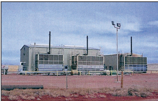
FIGURE 18 Typical CBM compressor station. Source: Wyoming State Geological Survey, 2001.
