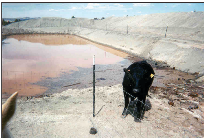
FIGURE 23 Photograph of cow in poorly fenced, unlined reserve pit, BLM land, northern New Mexico. Photo courtesy T. Blancett.
