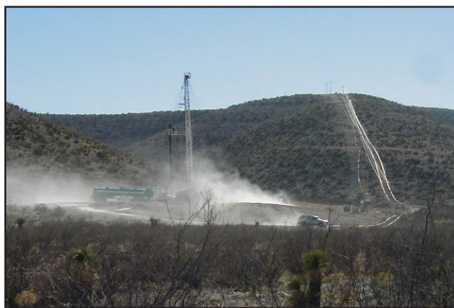
FIGURE 24 Drill rig near Carlsbad, New Mexico. Blowing dust is from vehicles driving on well pad and connecting roads.
